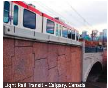
Light Rail Transit - Calgary, Canada
