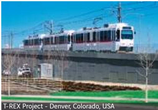
T-REX Project - Denver, Colorado, USA
